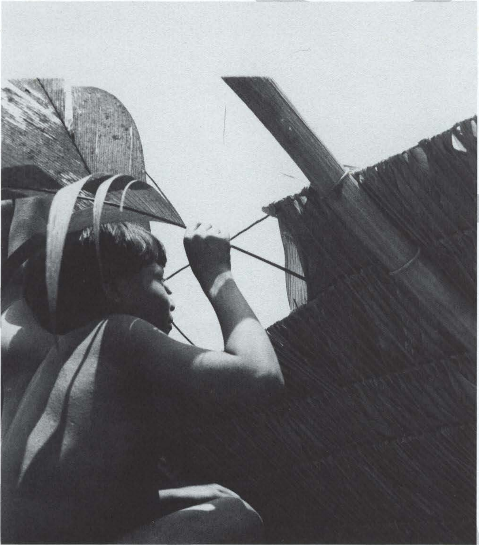
18. Thatching the shabono roof with leaves from the bisaasi kä hena plant.
